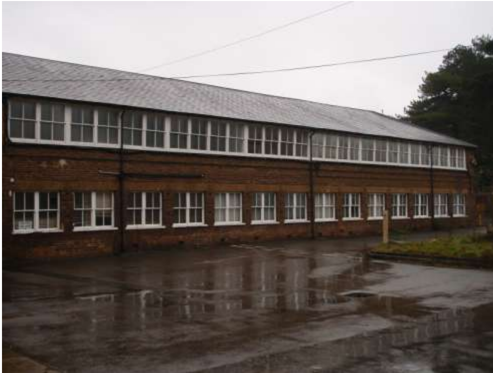
Plate 1. View of the listed Rag Room
